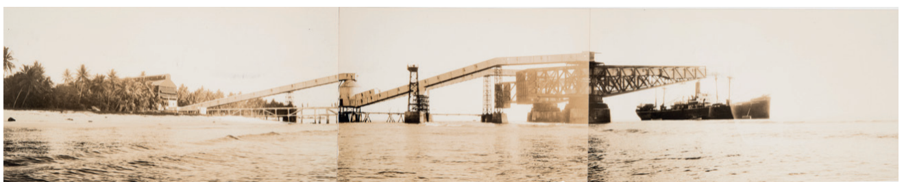
Fig. 3 Steel cantilevers and conveyor system on Nauru in c. 1932. Maslyn Williams Nauru Photographs, State Library of New South Wales, PXB 293, Image 116.
