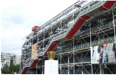
Fig. 2 Centre Pompidou by Rogers, Piano and Franchini.
