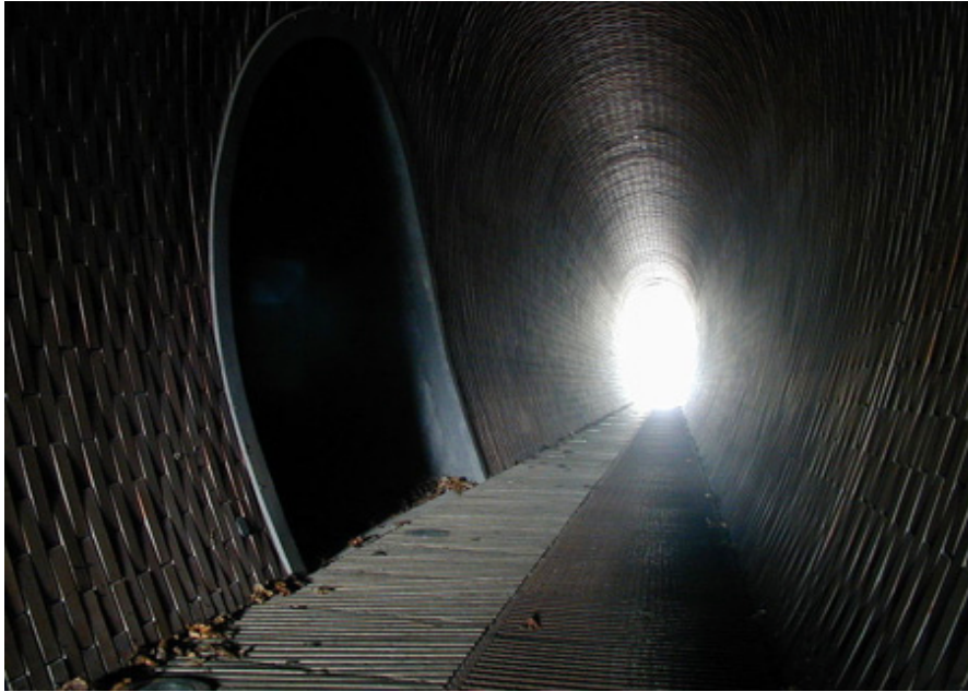
Fig. 4 Josef Pleskot, pedestrian tunnel in the Deer Moat, Prague Castle 2001–2002.
